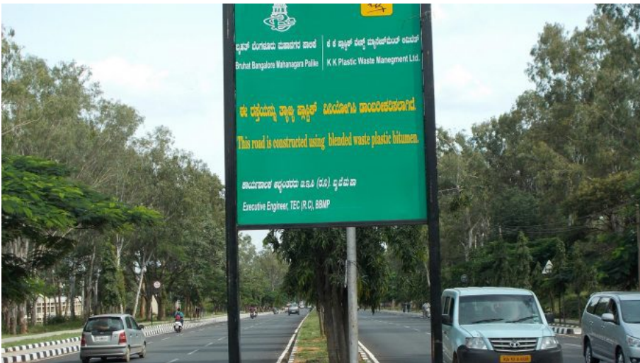
A road in Bengaluru constructed out of plastic waste. Source: KK PLastic Waste Management facebook page.
